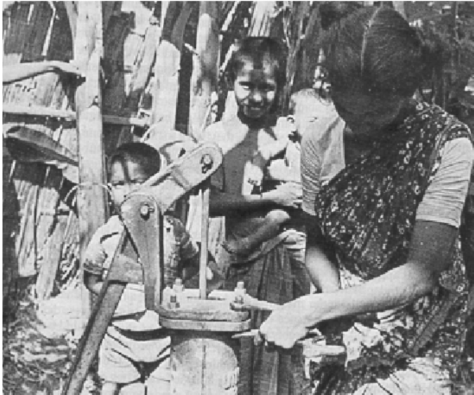
Figure 11. Participation of women in local maintenance: a woman caretaker repairs one of the many handpumps in Bangladesh (IRC photo by Akil Khan).
